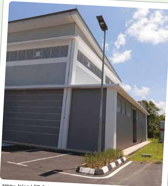
Lampu Jalan LED Solar di Residensi Kota Tinggi, Johor Solar LED Street Lights at Residensi Kota Tinggi, Johor
